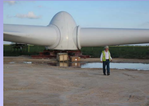
The blades "furrow or rotate" into the wind during extreme winds
